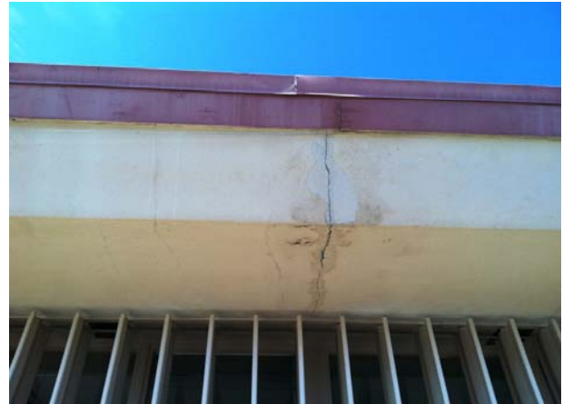
SBCA wing ( 116-120 + Library). Roof rated Poor Overall Condition, 15+ years old. Multiple issues, we recommend test and scan for possible retrofitting, and re-roofing as soon as possible.
