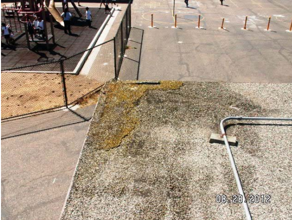
SBCA wing ( 116-120 + Library). Roof rated Poor Overall Condition, 15+ years old. Multiple issues, we recommend test and scan for possible retrofitting, and re-roofing as soon as possible.
