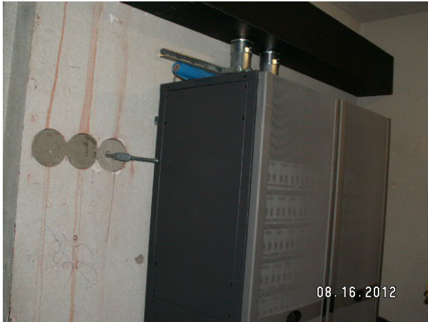
Existing Lighting Control Panel. Project includes an upgrade to the system
